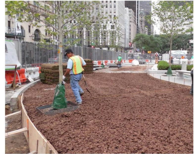
Structural Soil Installation
