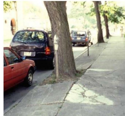
Trees Planted in Limited Soil Volumes Struggle to Survive and Often Damage Adjacent Sidewalks
