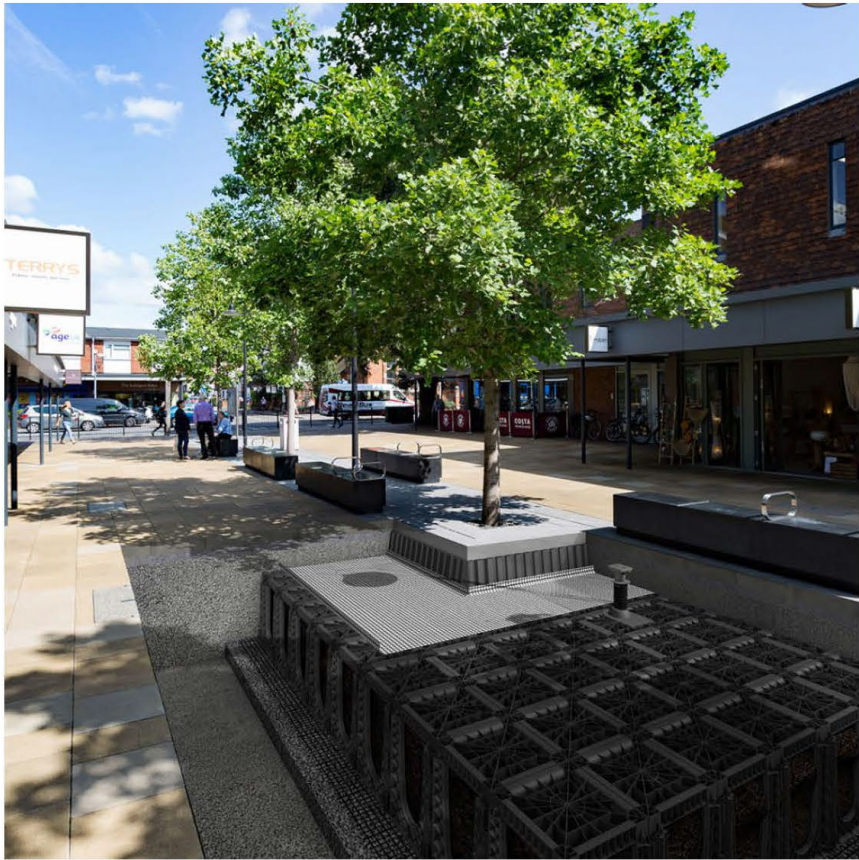
GreenBlue Urban Soil Cell Pavement System Install
